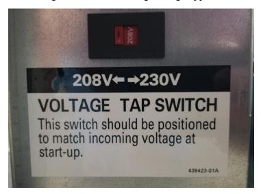
It is also possible to add a transformer in the field, for single phase 208-230 units that do not come from the factory with one installed. This is particularly helpful in replacement applications where the available circuit does not have a neutral and it may be difficult or costly to add the neutral wire.
