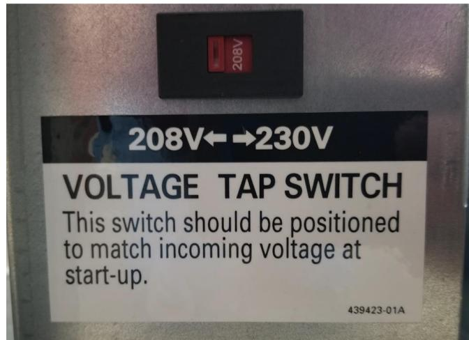
When installing a unit that includes a center tap transformer, it is important that the voltage tap switch be moved to the correct voltage based on the voltage being supplied to the unit, either 208 or 230.
